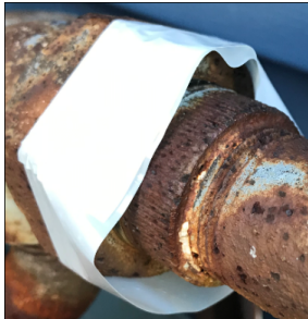
Method 1: First apply to larger diameter then crimp down remaining adhesive with hand
