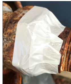
Method 2: Use slight (1/4”) overlap if wider application is necessary
