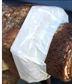
Method 1: First apply to larger diameter then crimp down remaining adhesive with hand
